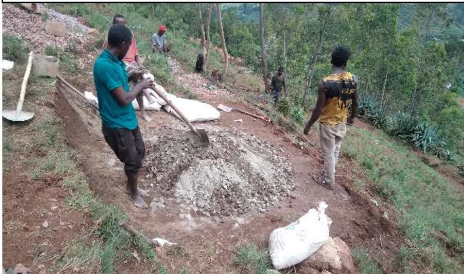
Mix with water (use jerrycan for water to control closely the workability)
