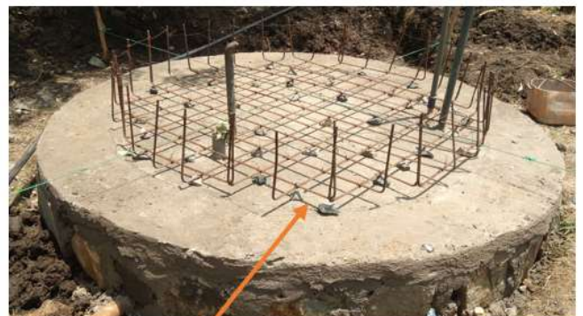
20mm to 30 mm crushed stone spacer
