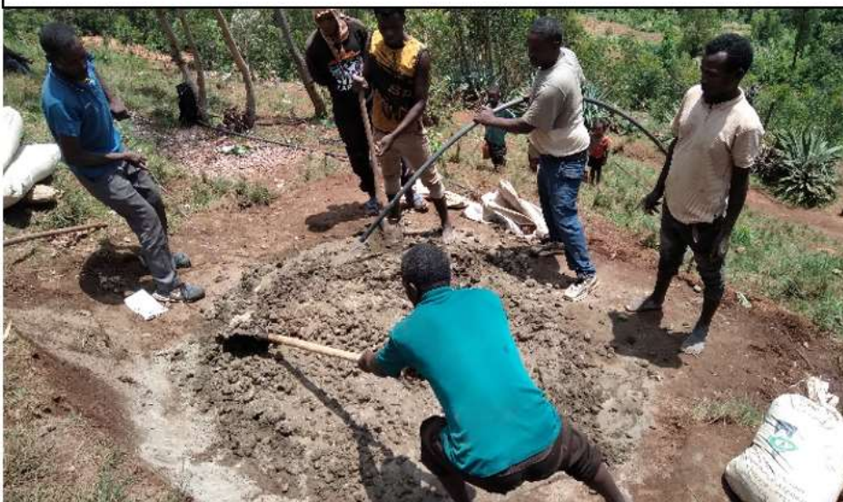
Mix with water (use jerrycan for water to control closely the workability)
