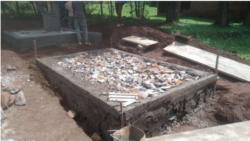
Wash table masonry foundation work on going:
