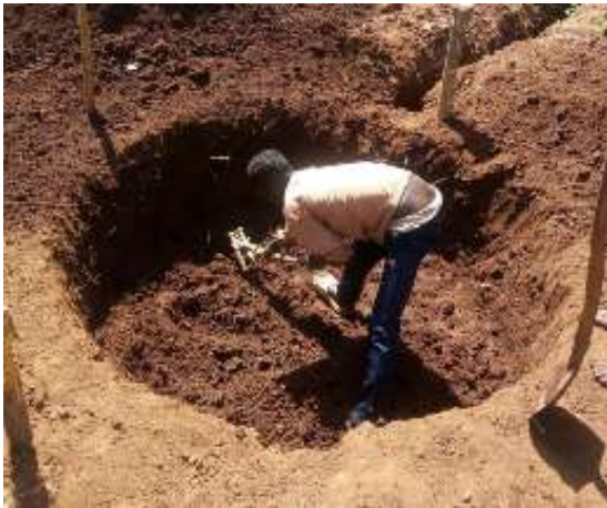
Reservoir foundation digging:
