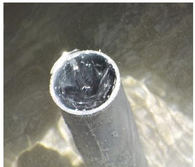
Figure 1: Shaft spillway discharge (from Design of small dams, Bureau of reclamation, 1987)
