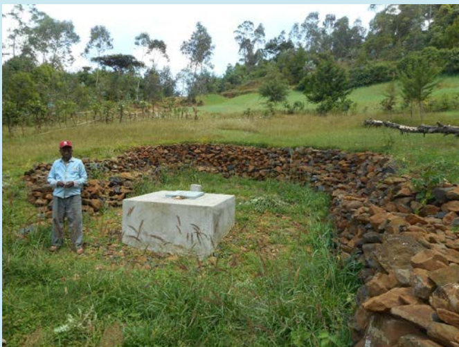
Spring Outside View: Close protection and catchment perimeter fenced (against animals)
